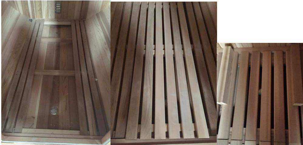
Floor Part A shall be fixed to the staves with screws.
